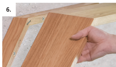
6. Align the shelf directly to the mounting strip
