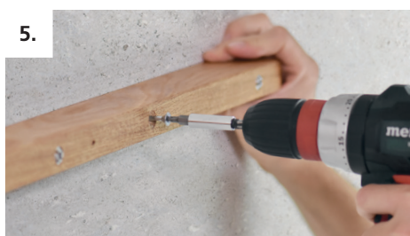
5. Align the mounting strip and fasten it to the wall
